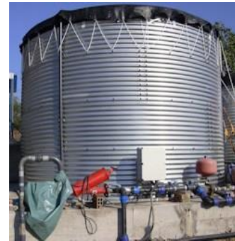
Vasca o Cisterna
